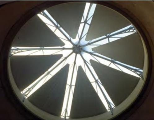
There is a variety of shading skylight systems consisting of standard hardware for sloped, incline and flat glazing – the ability to provide custom complex engineered shades for any shaped skylight is possible. Shades are available in gravity drop utilizing roller gliders in tracks, as well as bottom up, with single or double motor and special tension systems for any overhead glazing.
